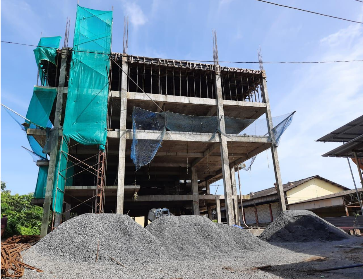
Present status project site.
