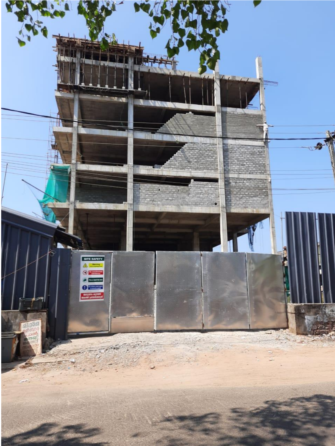
Present status project site.
