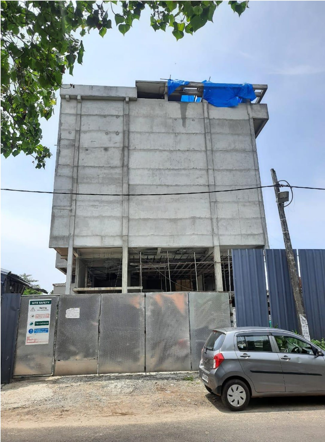
Present status project site.
