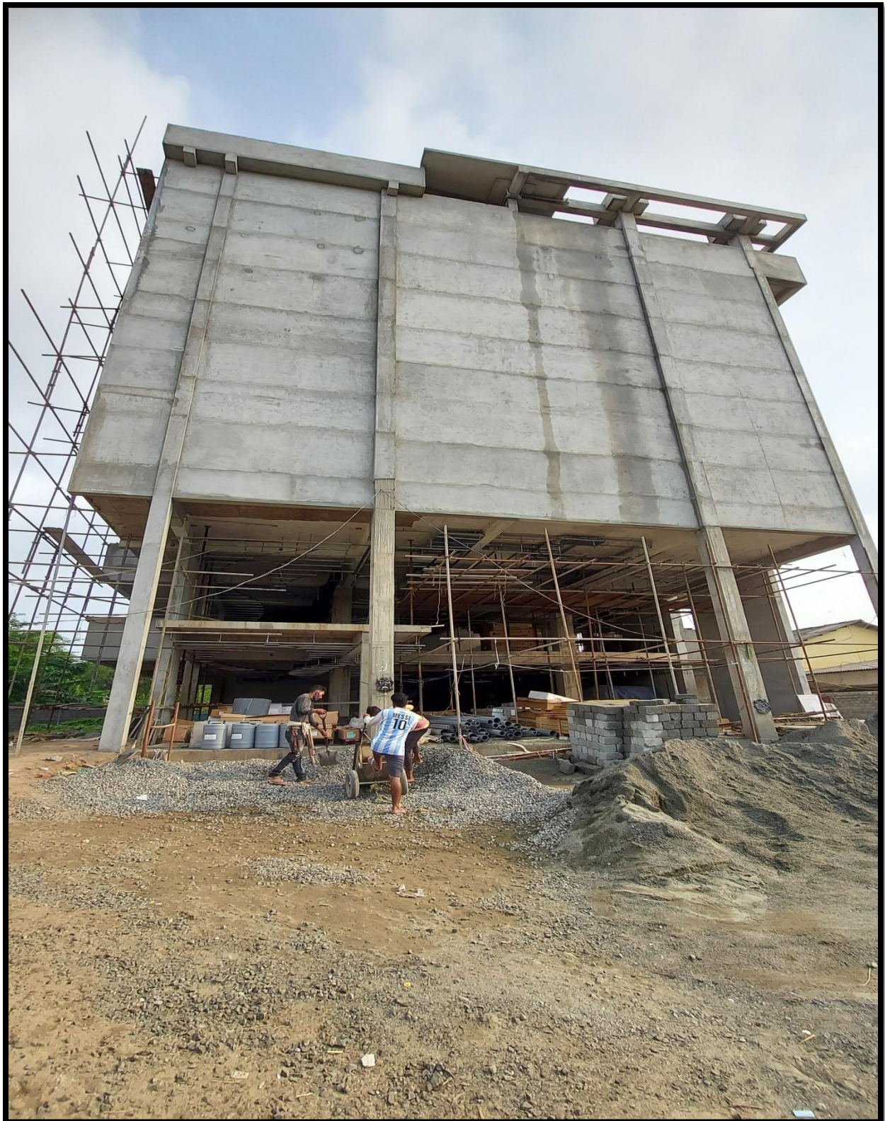
Present status project site.
