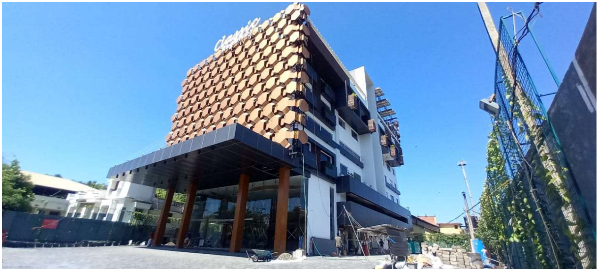
Present status project site.
